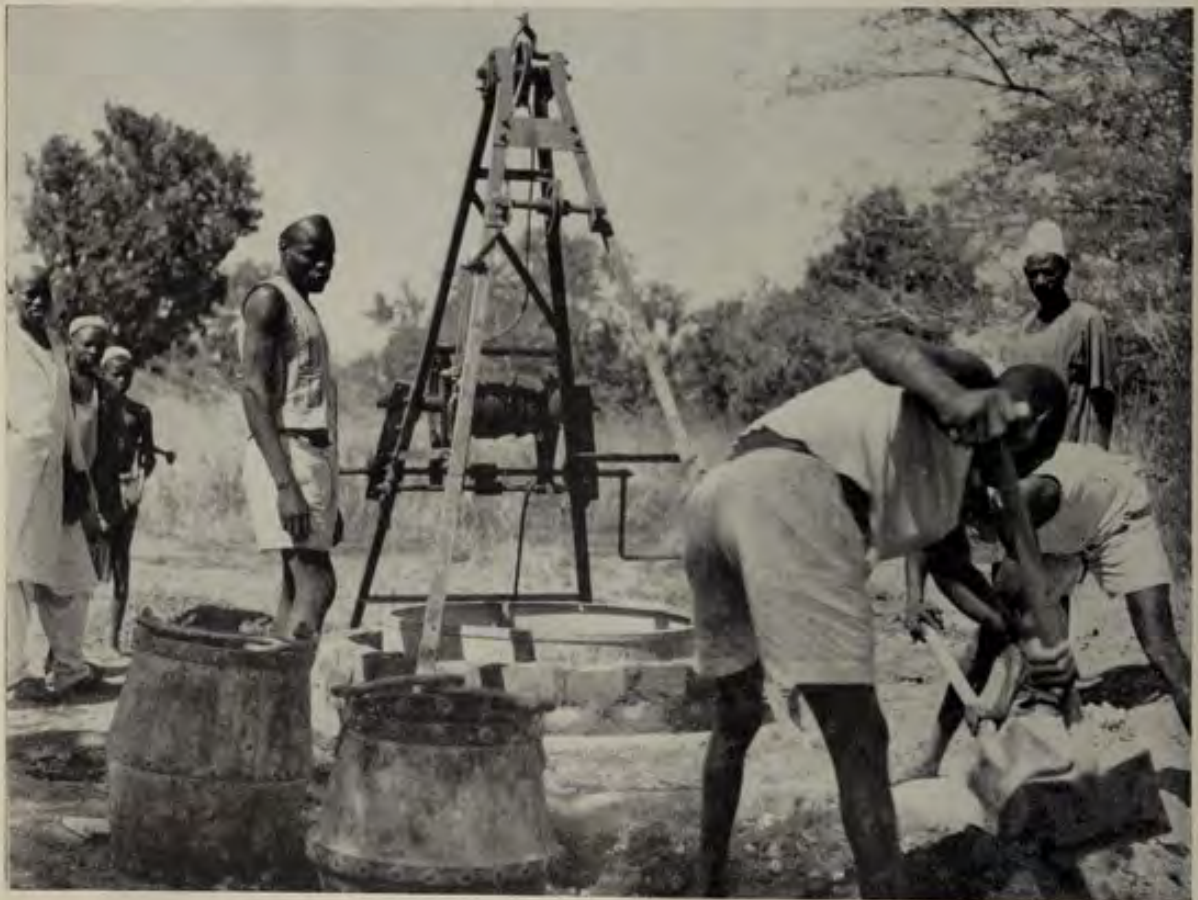
Well sinking at Gwoza settlement, Northern Cameroons.
