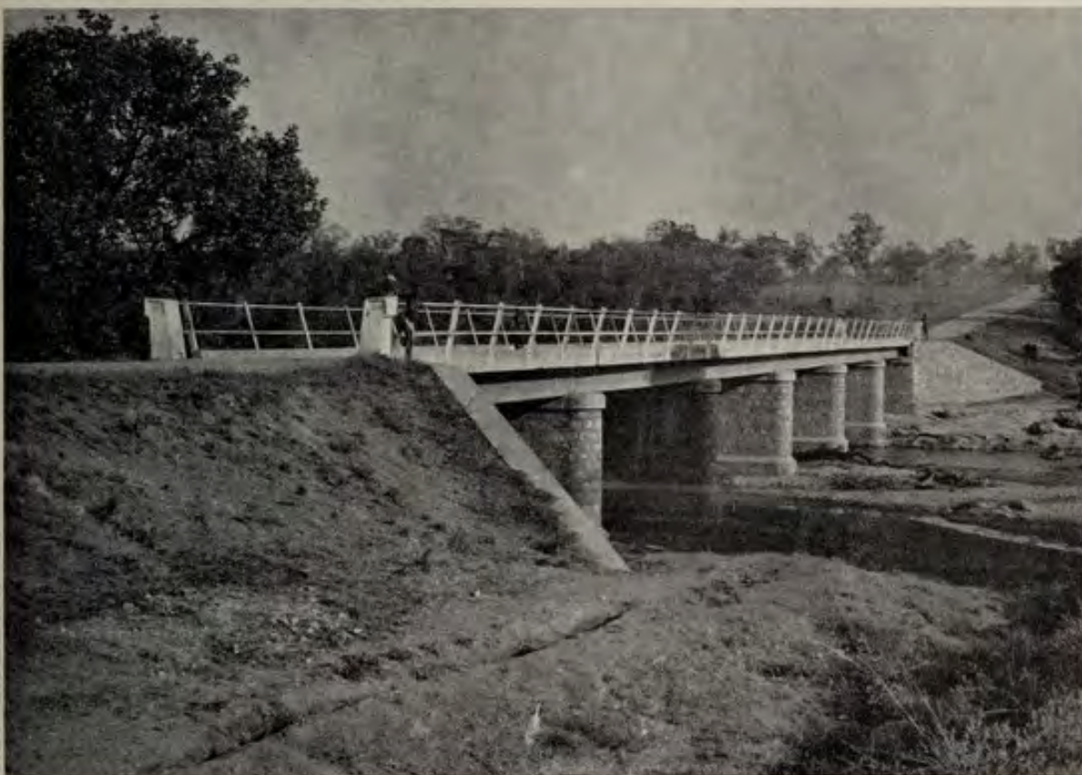
New bridge construction, Berli-Serti Road, 1957.
